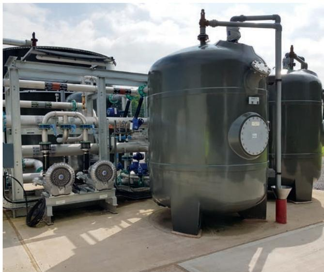
FilterClear Pre-filtration for Desalination
