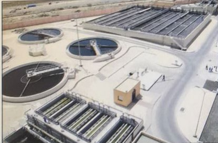
■ The Tubli WPCC ... upgrade underway
