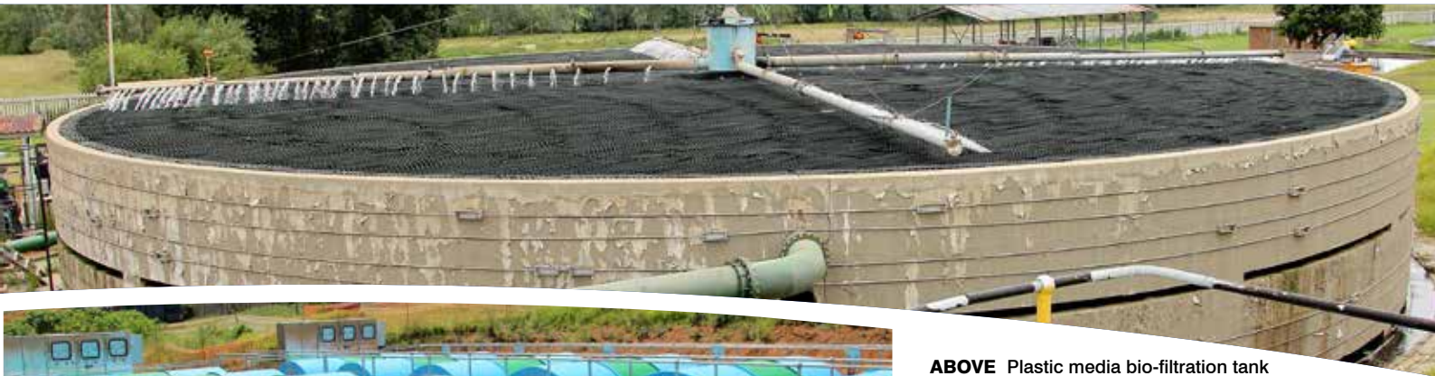
ABOVE Plastic media bio-filtration tank LEFT HYBACS installation at Tsakane
