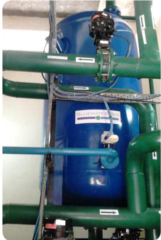
The biological treatment plant was commissioned at the beginning of May 2013 and the FilterClear™ plant was commissioned at the beginning of June, operating at a loading velocity of 24 m/h. Figure 1 shows the daily performance of the FilterClear plant since commissioning.
