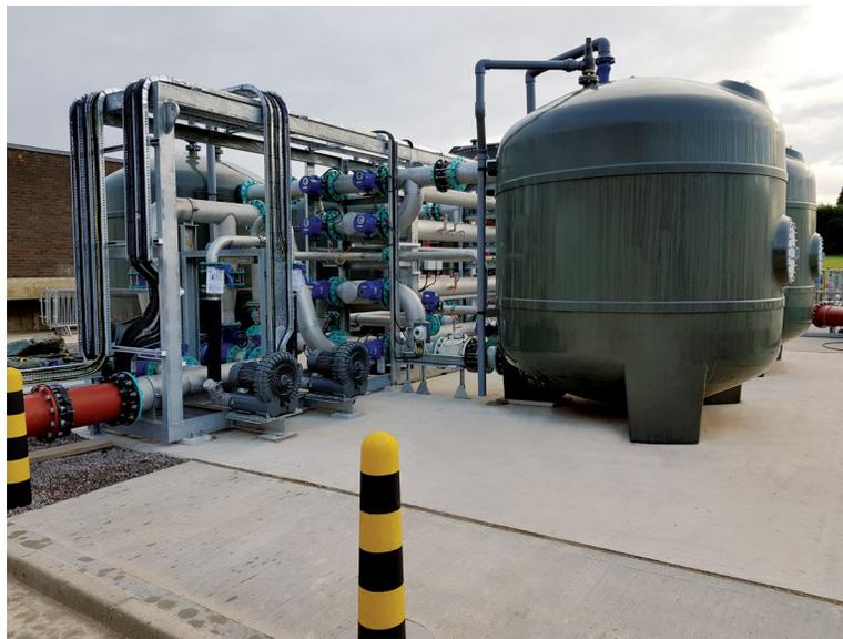
*Fully automated 4v2800 FilterClear plant installed at Ledbury WWTW*
